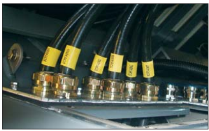
Cables can be safely inserted into the equipment cabinet module. A ShrinkTrak heat-shrinkable tubing marker is used for labelling.
