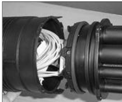
41. Fit the cover onto the closure.
