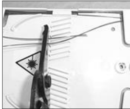
11. Cut the fibres on the opposite side of the fins.
