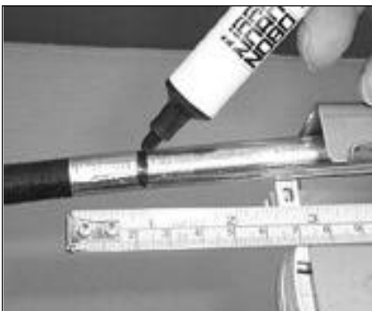
25. Mark the foil 20mm from position 'A'.
