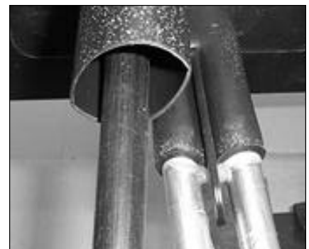
51. Insert cable in to the port.
