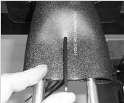
37. Separate the cables and insert the branch clip provided.
