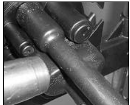
69. Recover the heatshrink on to the cable.
