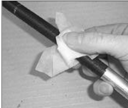
20. Clean the abraded area of the cable using an IPA wipe supplied.
