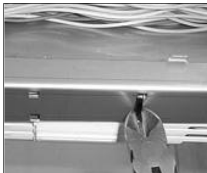
71. Cut the cable ties securing the fibre unit to the basket.
