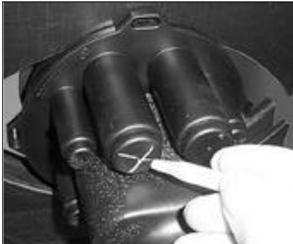
46. Identify which port will be used for the spur cable.
