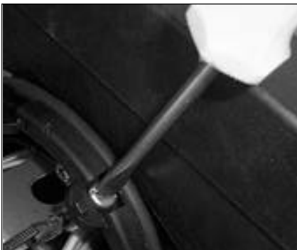
67. Secure the central strength member using the fixings provided. Refer to steps 28 to 30 for details.
