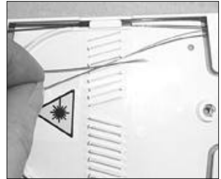
12. Splice the fibres using standard procedures
