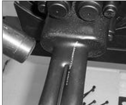
38. Recover the heatshrink onto the cable.
