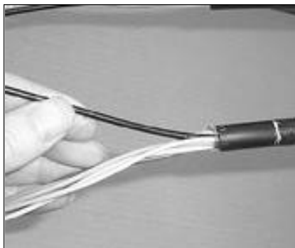
26. Ensure the central strength member is separated from the fibre units.
