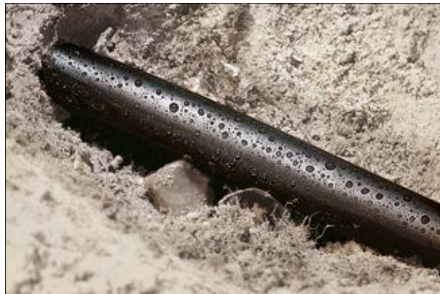
TREDUX HA47 - application below ground.
